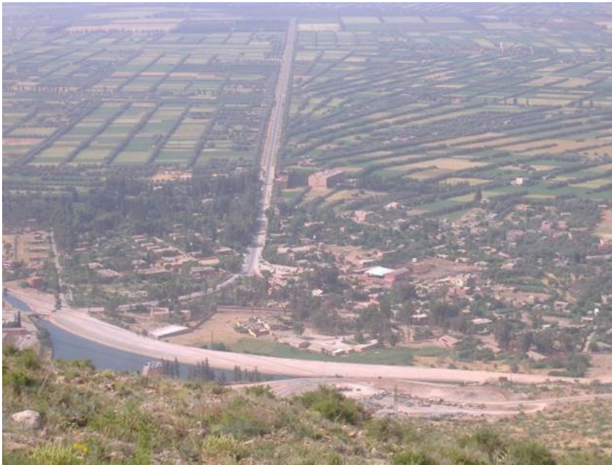
Fig. 2. Tadla large irrigation scheme in Morocco (photo by Caron, 2006).
