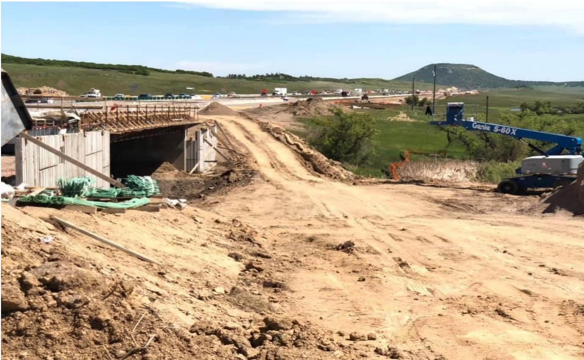
I-25 Mind the Gap Project Progress
