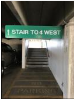
Finding 298035 Additional Photo
