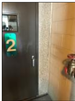
Finding 298020 Additional Photo
