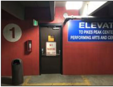
Finding 297982 Additional Photo
