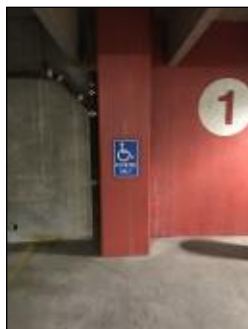
Finding 297983 Additional Photo
