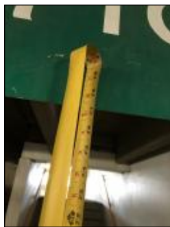
Finding 297996 Additional Photo
