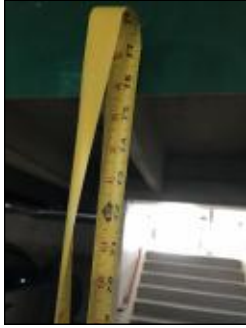
Finding 297987 Additional Photo
