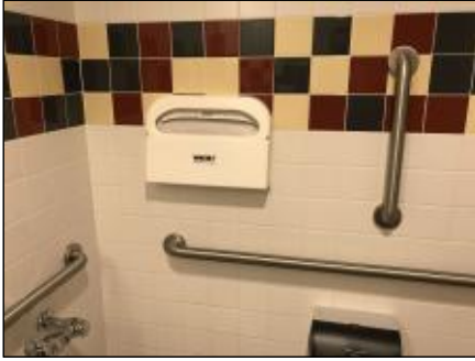
Finding 299280 Additional Photo
