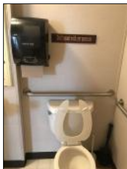
Finding 299294 Additional Photo
