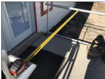
Finding 299235 Additional Photo
