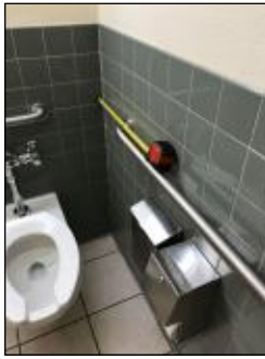
Finding 299251 Additional Photo
