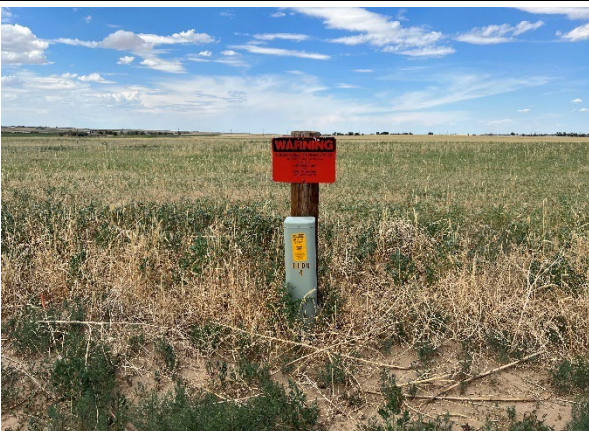
Photo 5: Buried Utility lines on the southern portion of the Subject Property.
