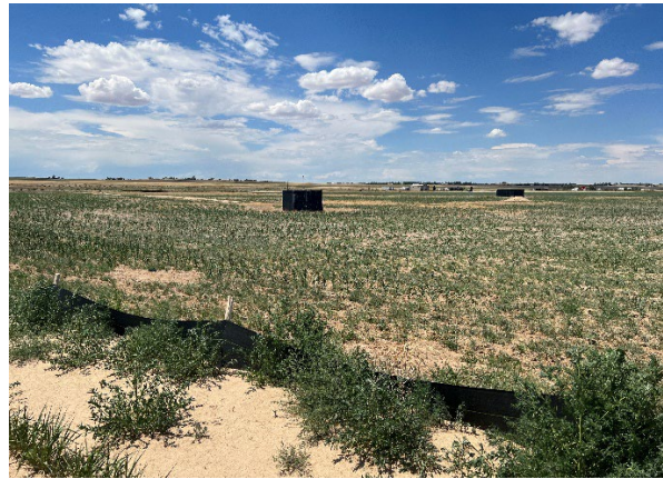
Photo 10: Pumping Equipment to the northwest of the Subject Property.
