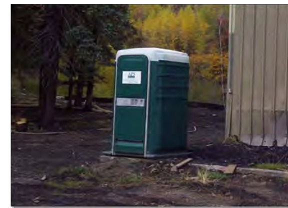
Photograph GH-3. Locate portable toilet facilities on level surfaces away from waterways and storm drains. Photo courtesy of WVE.
