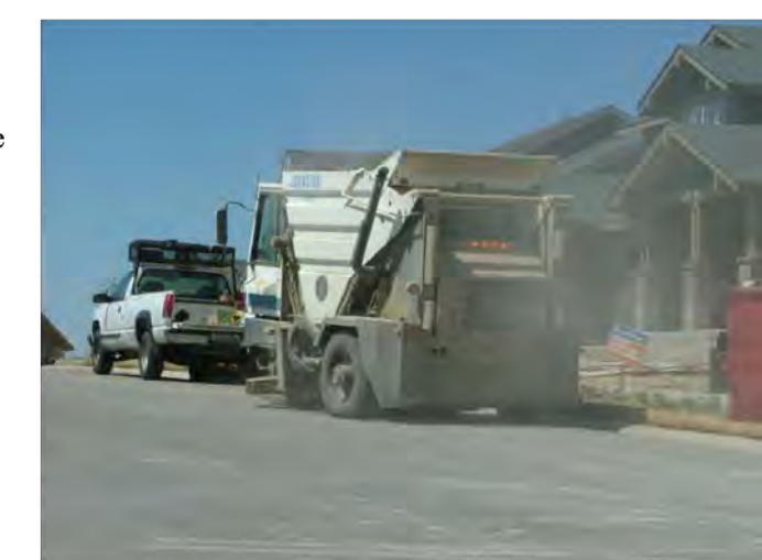
Photograph SS-1. A street sweeper removes sediment and potential pollutants along the curb line at a construction site. Photo courtesy of Tom Gove.
