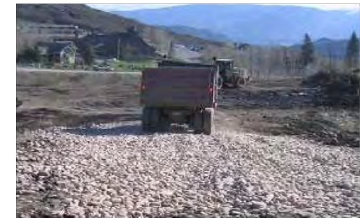
Photograph VTC-1. A vehicle tracking control pad constructed with properly sized rock reduces off-site sediment tracking.
