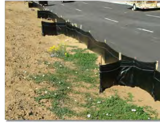
Photograph SF-1. When silt fence is not installed along the contour, a 'J-hook' installation may be appropriate to ensure that the BMP does not create concentrated flow parallel to the silt fence. Photo courtesy of Tom Gore.
