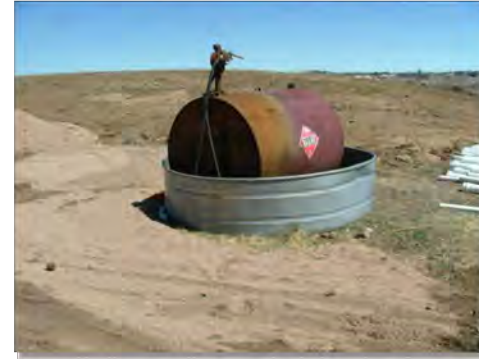
Photographs GH-1 and GH-2. Proper materials storage and secondary containment for fuel tanks are important good housekeeping practices. Photos courtesy of CDOT and City of Aurora.
