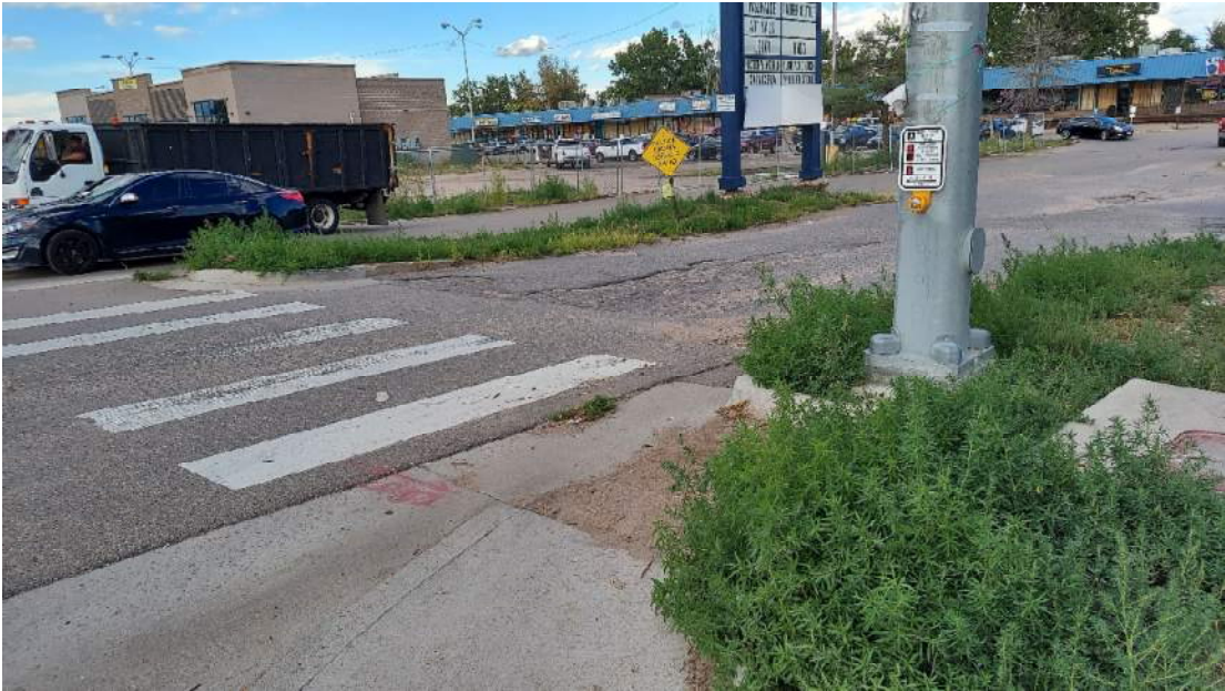
P1. 53 rd Place intersection at Sheridan Boulevard, east side of the roadway.
