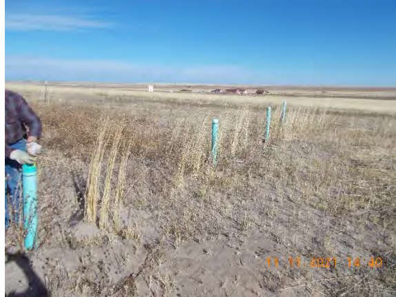
Inspection Ports at south end of STA
