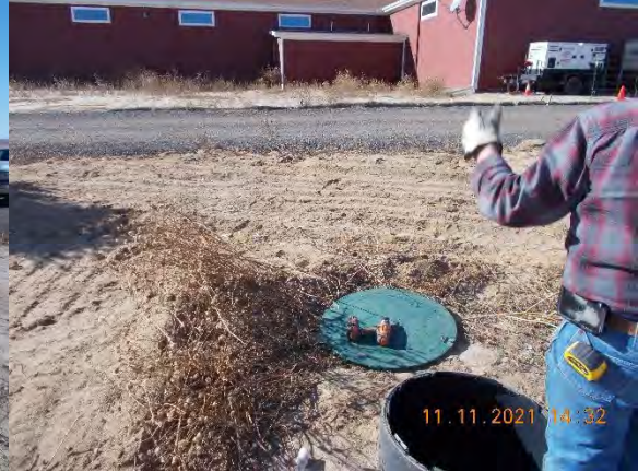
Looking west from tank to building
