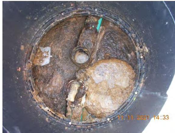
Access port for tank – Before Pumping
