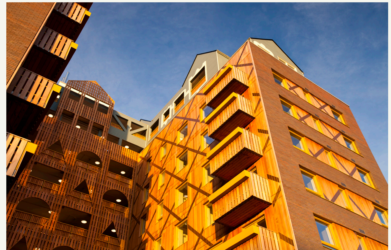
Riverside One, in Teeside, UK, is an exceptional green building whose individual housing units have a low carbon footprint. The whole block is heated by a biofuel boiler. During construction it used recycled oil rig pipes for piling, the concrete was mixed with recycled aggregate, super insulated with earth wool, it uses grey recycled water to save water, locally sourced timber, the electricity for the building is sourced from renewable sources and the building incorporates Swift bird boxes and bat boxes. © Global Warming Images / WWF
