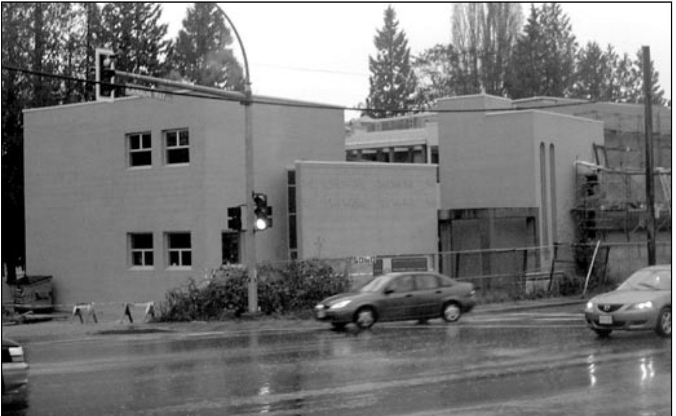
Burnaby Mosque, Under construction
