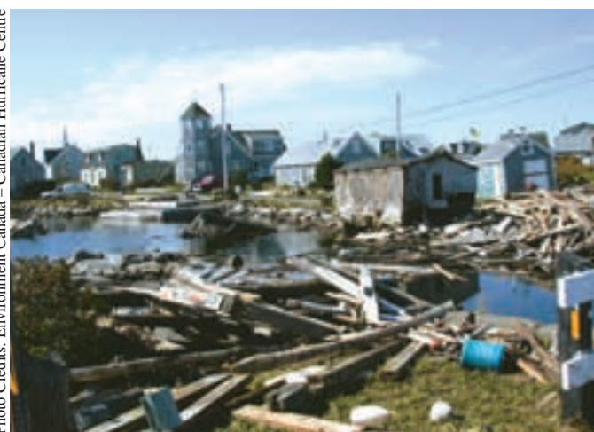
Hurricane Juan damage at Prospect, Nova Scotia, 2003
