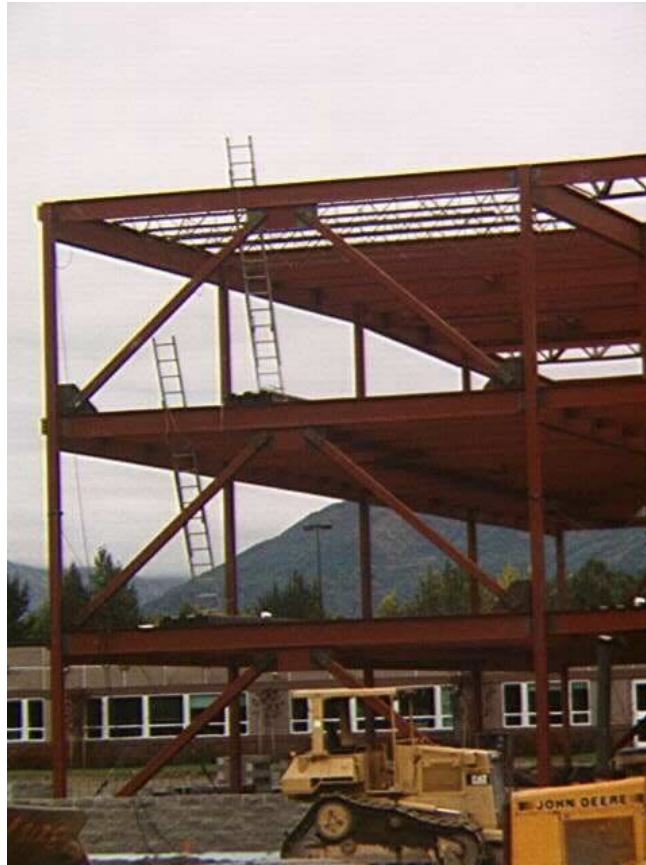
Figure 6.19. Example of a braced steel-frame.
