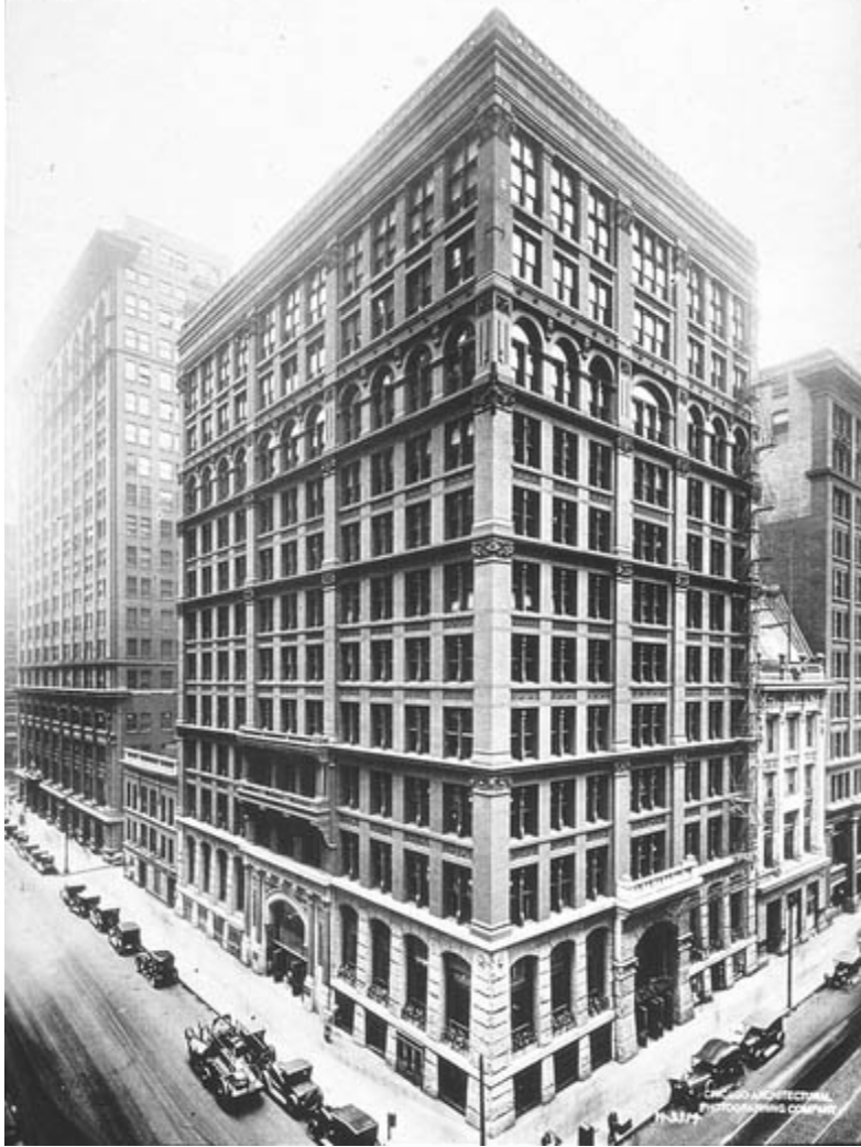
The Home Insurance Building – Chicago, IL, 1885, an early skyscraper
