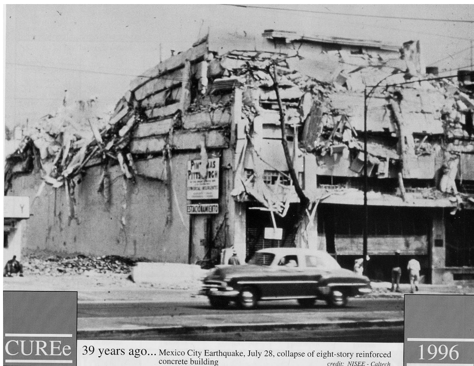
Figure 6.14. Collapse of an 8-story non-ductile concrete moment-resisting frame building in Mexico City from the 1957 Acapulco earthquake.
