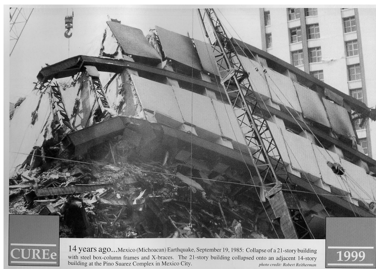
Figure 6.46. Close-up of the left tower in Figure 6.45.
