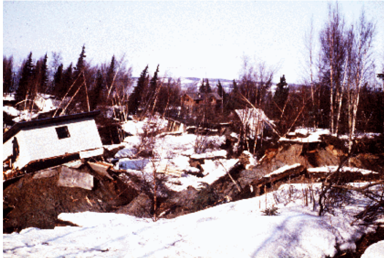
1964 Alaska Earthquake, Turnagain Heights
