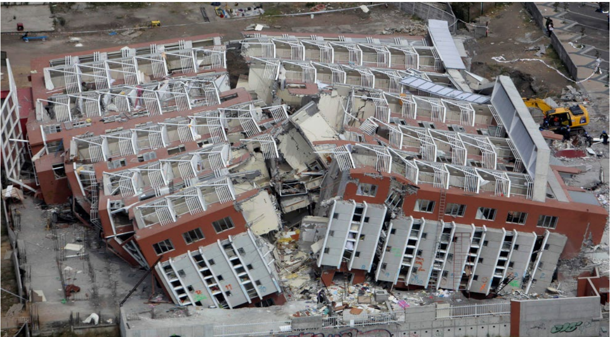
Shear failure in a new 25-story shear wall building in the 2010 Maule earthquake
