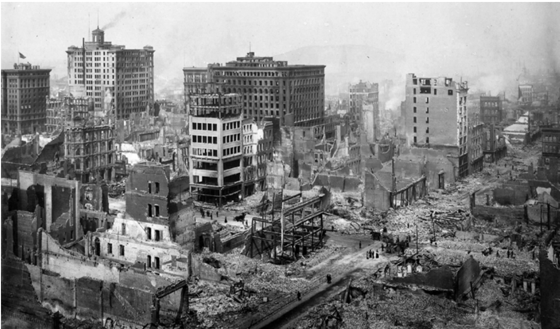
Steel frame buildings in downtown San Francisco performed well in the 1906 earthquake.
