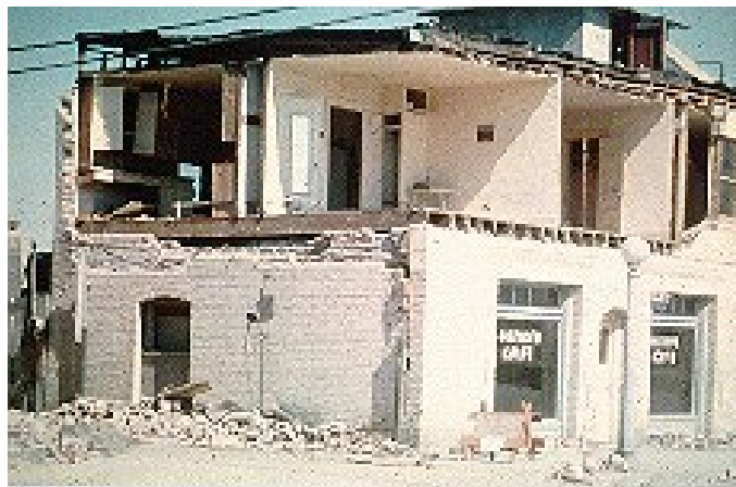
Figure 6.23. Example of an unreinforced masonry building (URM).
