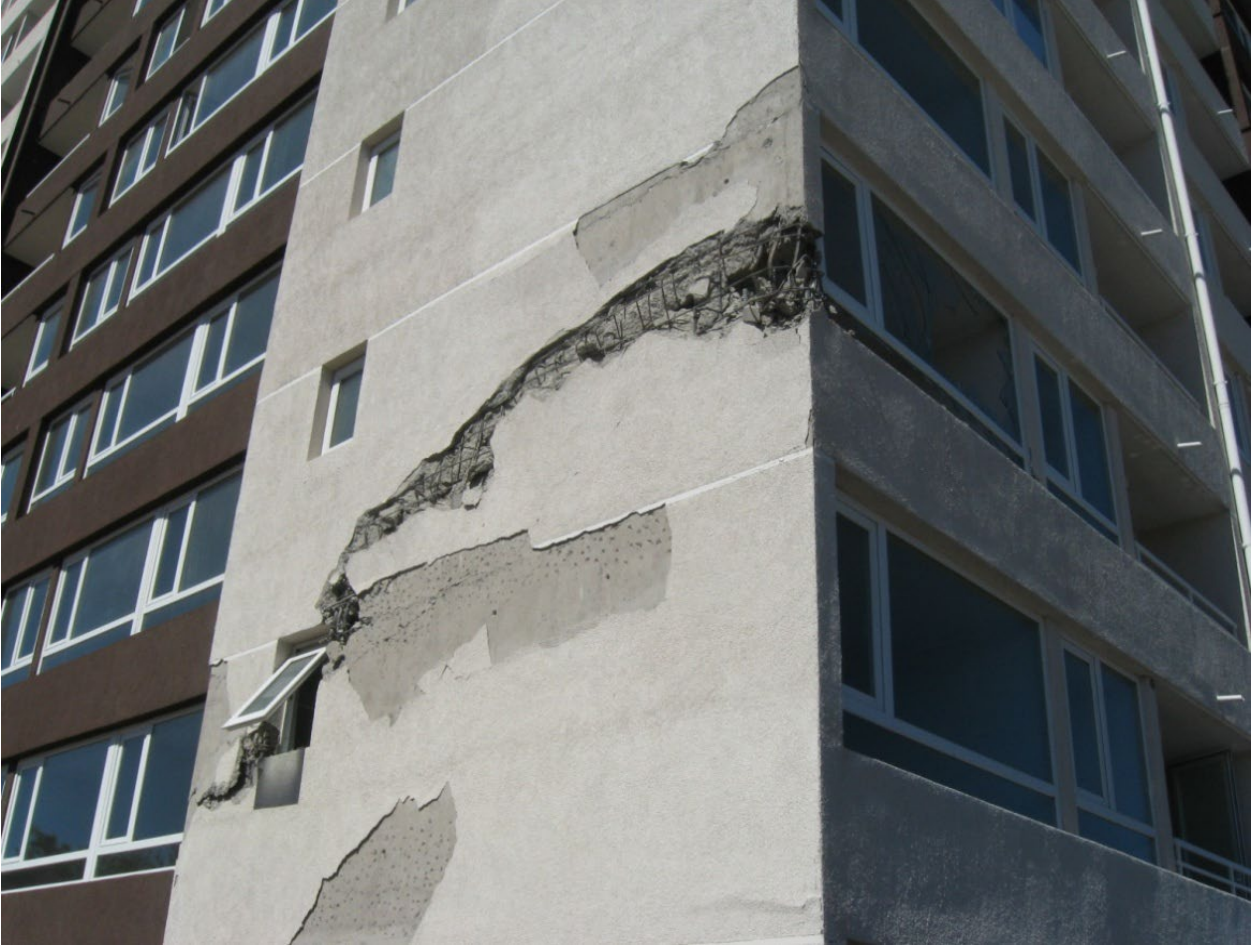
Shear failure in a new 25-story shear wall building in the 2010 Maule earthquake
