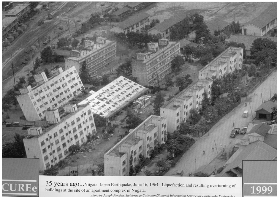
Figure 6.3. Japanese concrete shear-wall apartment buildings after the 1964 M 7.2 Niigata earthquake. Despite the fact that the foundations of the buildings failed due to liquefaction, the building structures were undamaged and the buildings were later jacked back to an upright position and they were reoccupied.
