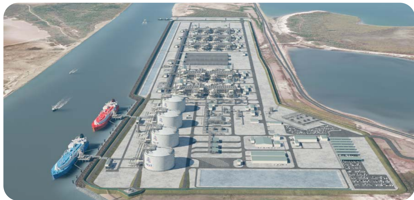
NextDecade Rio Grande LNG facility – Brownsville, Texas. Courtesy of NextDecade Corporation
