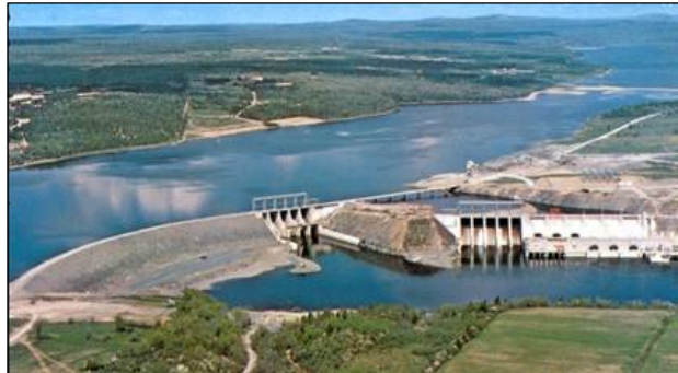
Figure 1. Mactaquac Dam, Keswick Ridge, NB (from Agora, 2008)
