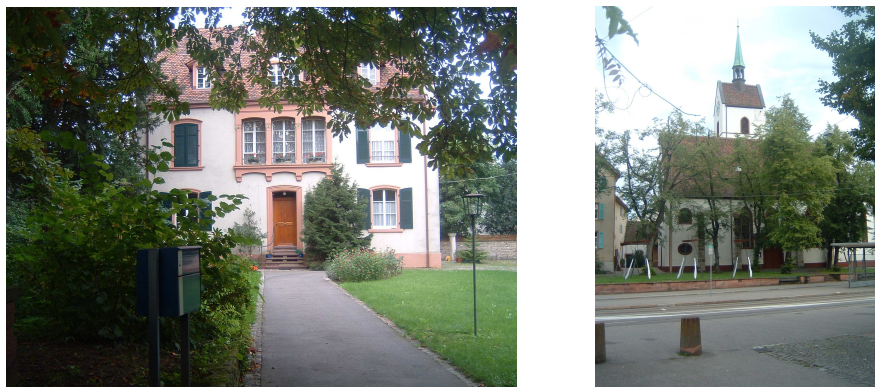
Figure 1: The parish residence and church in Riehen
