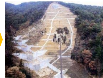
Completion of restoration works
