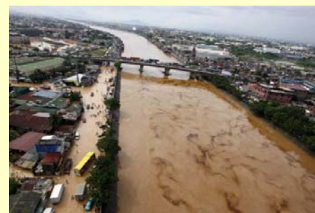
Manggahan floodway, Japan supported for its construction
