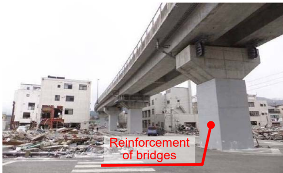
Condition of a bridge after the Great East Japan Earthquake (seismic reinforcement was completed)
