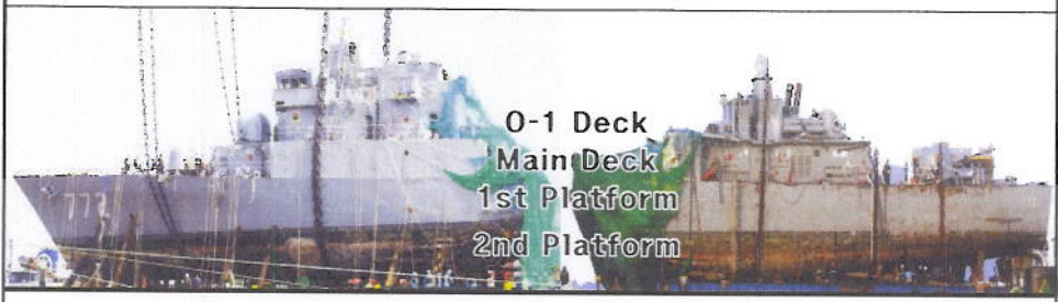
전체 모습 Overall structure
