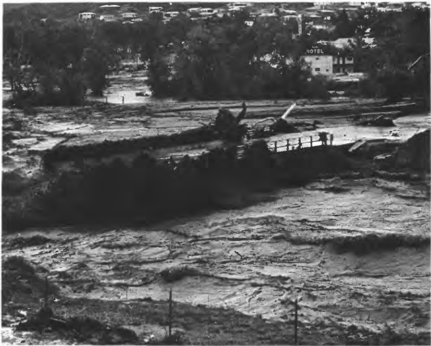
FIGURE 9.—Bridge on approach road from Castle Rock to Interstate Highway 25 destroyed by East Plum Creek. Denver Post photograph by William Peters.
