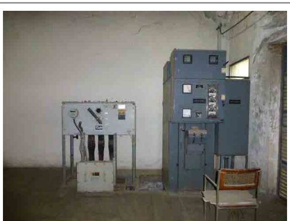
Figure 8.1.1-1 Existing Changeover Switch and Energy Meter Panel
