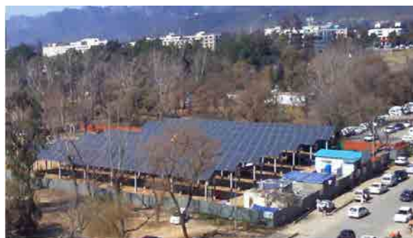
Solar System at PEC
