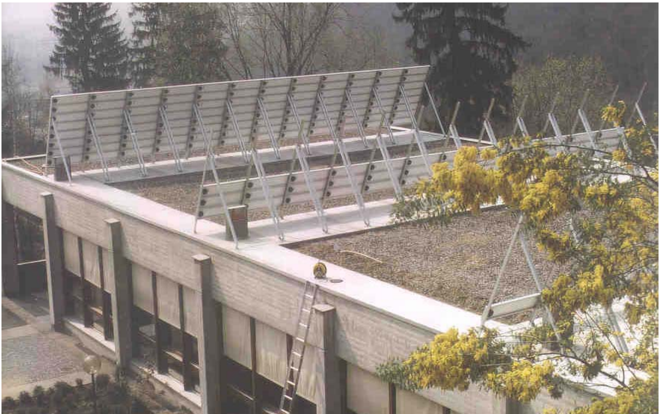
Figure 2: rear view of the TISO 10 kW plant during its installation (1982).
