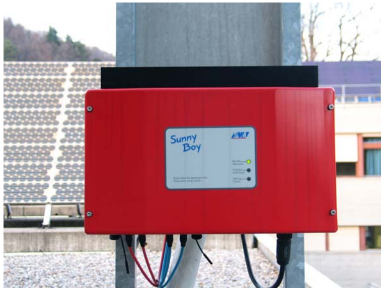
Figure 52: Sunny Boy 2500 inverter connected to one field of the TISO plant.
