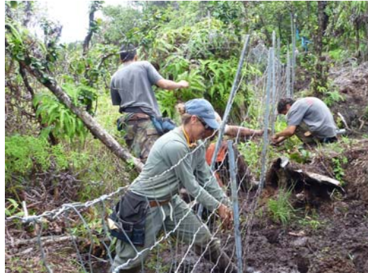
Installing fence in East Maui's watershed
